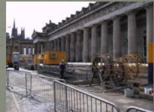
Work at Site
